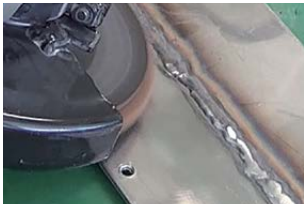
Removing blue weld discoloration
